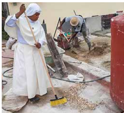
Sisters from the “Siervas de María” Convent renovating the roof.
